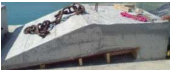
Figure 4 Wedge-shaped concrete block anchor
