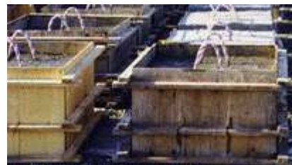
Figure 5 Square concrete block anchor
