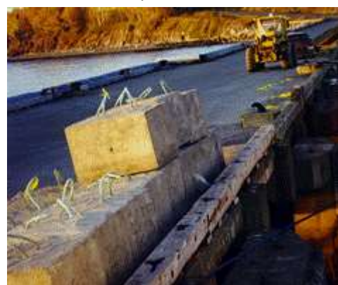
Figure 32 Anchor blocks loaded on dock
