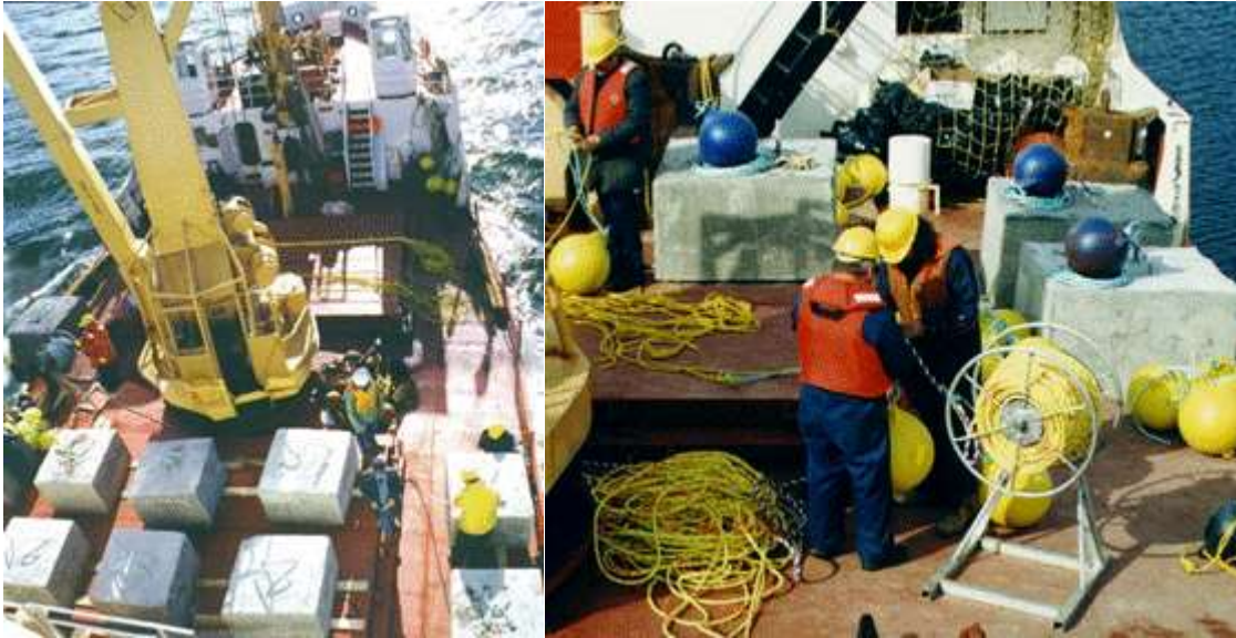
Figure 44 Transporting and preparing the concrete anchors and longline ropes loaded onto a 60m ship
