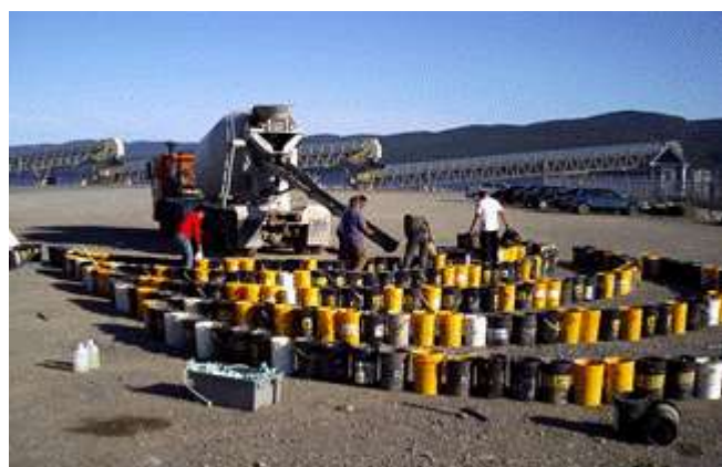
Figure 17 Production of compensation ballast weights
