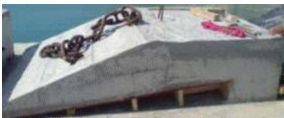
Figure 4 Wedge-shaped concrete block anchor
