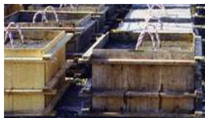
Figure 5 Square concrete block anchor
