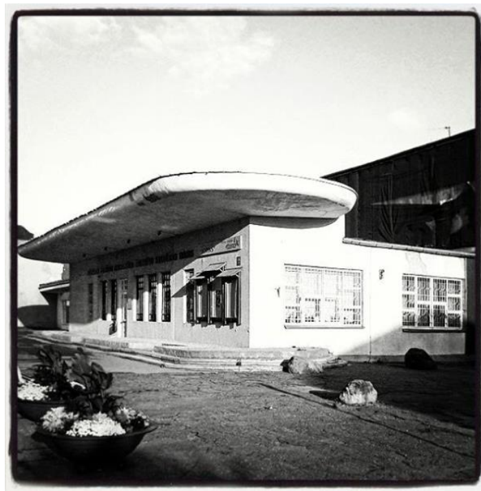
Cinema in Rēzekne, 1961 Demolished in 2015
