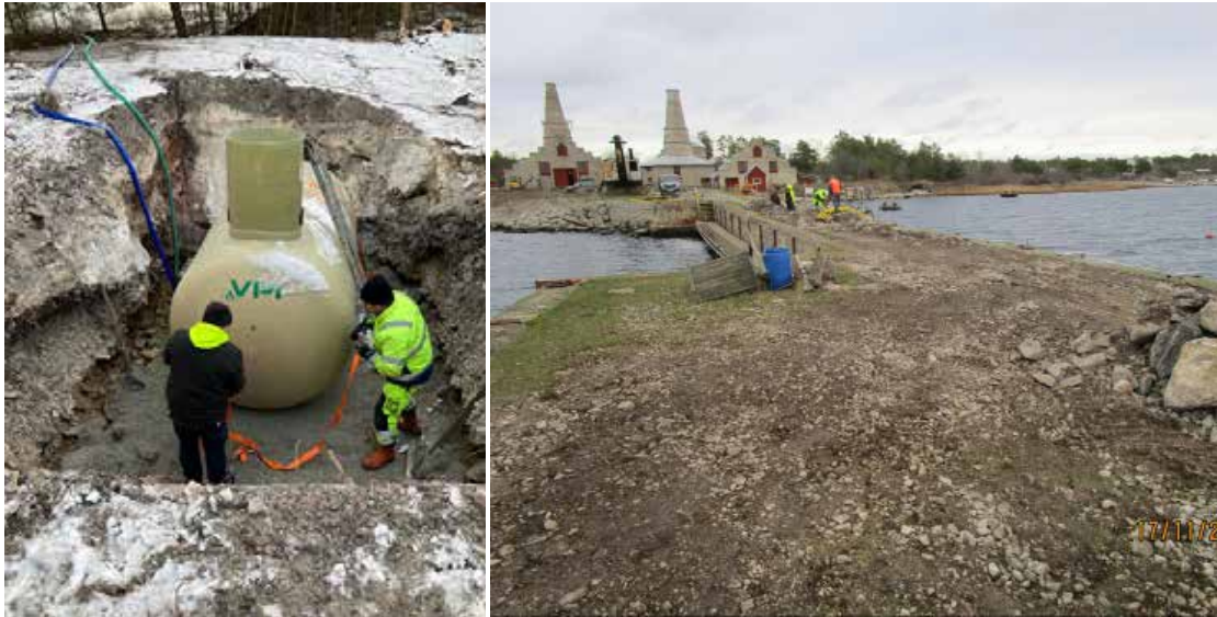
Pictures 45. Installing the septic waste tank and picture 46. Excavation work on quay. © Leif Ortman
