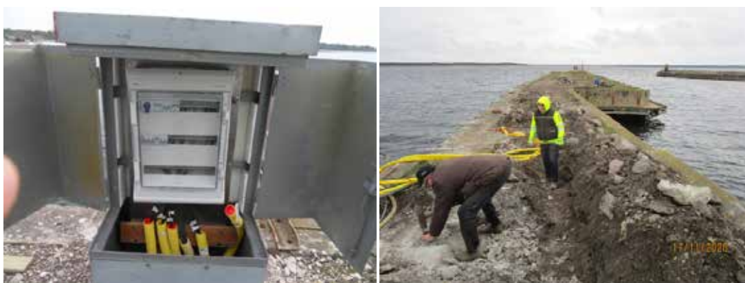
Pictures 35 and 36. The Sub-fuse box on quay and cable installations. © Leif Ortman
