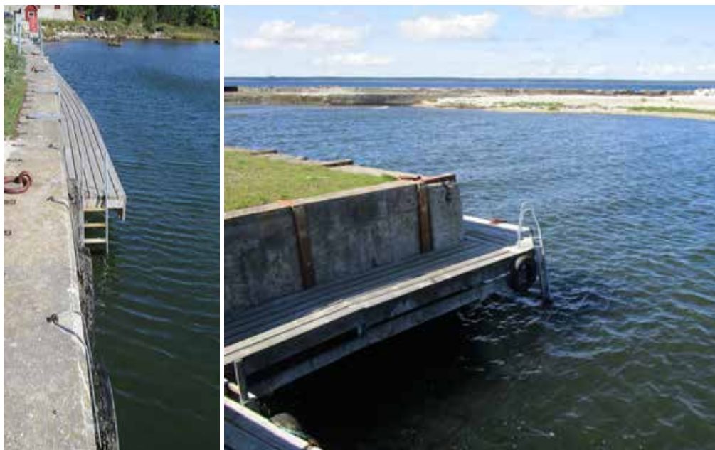
Pictures 41 and 42. The safety-ladders from water to the walking deck. © Leif Ortman
