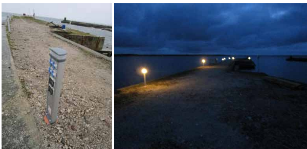
Pictures 35 and 36. The Sub-fuse box on quay and cable installations. © Leif Ortman
