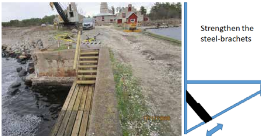
Pictures 39 and 40. Part of the renewed walking decks and new stairs up to quya from the walking deck and illustration of the strengthening measure. © Leif Ortman
